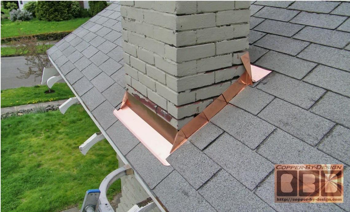
**(e)** You may want to add a little caulk in the corners to help seal them together, but if it is flashed right it should not be needed. There should be some copper from the upper flashing to be bent over the corners to seal them. I included some clear caulk in a small syringe.
